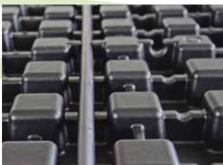
Slotting the dripperlines into place. The lines are then connected to the control system.
