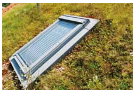
This roof with a pitch of approx. 5° is drained using a gutter and does not yet require any special measures.
