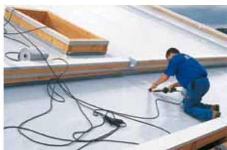
The roof area to be greened is sealed with rolls of waterproofing membrane that have been tested for their root-resistance in line with FLL procedures.
