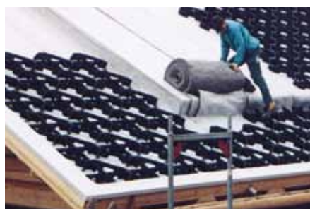
Once the area has been covered with the Protection Mat WSM 150, the Georaster® elements are installed, starting from the bottom up.
