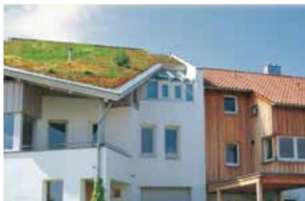
This semi-detached house near Tübingen, Germany, provides a contrast between different types of design. Wooden and rendered facade, tiled and green roof.
