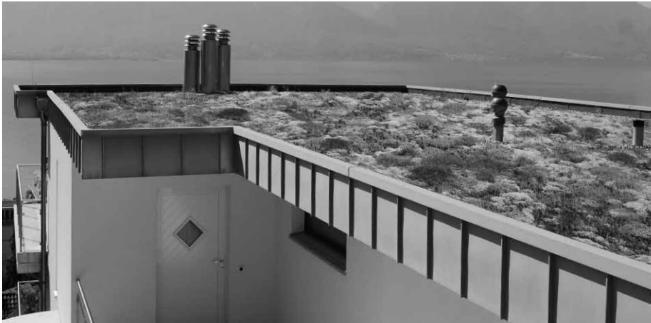
Extensive Green Roof
