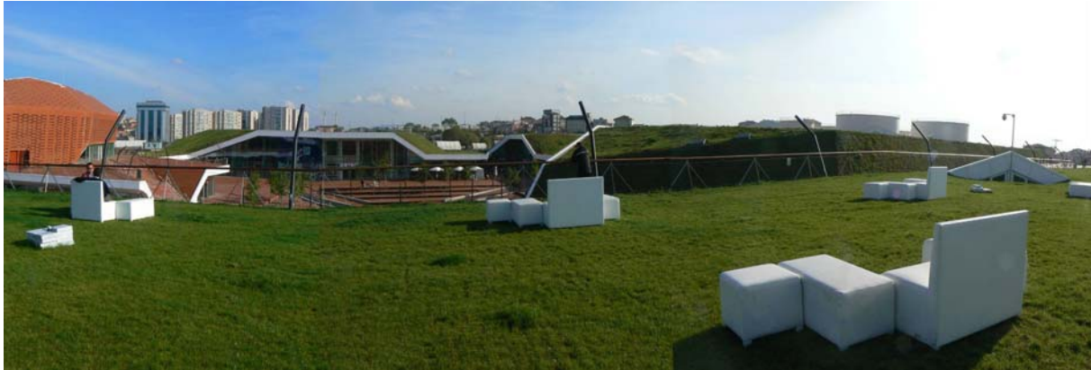
Image 4: A part of the roof area has been developed accessible and invite you to linger
