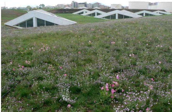
Image 7: Already after a few weeks a green carpet covered the roof landscape.
